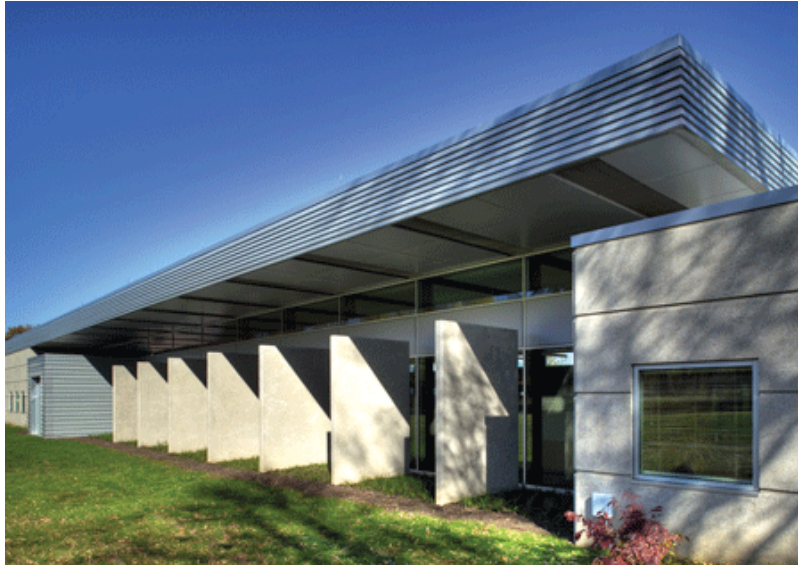
Ten-foot-tall precast vanes jut out at intervals on the western side of the building, allowing views of a natural wooded ravine while blocking out harsh sunlight.
